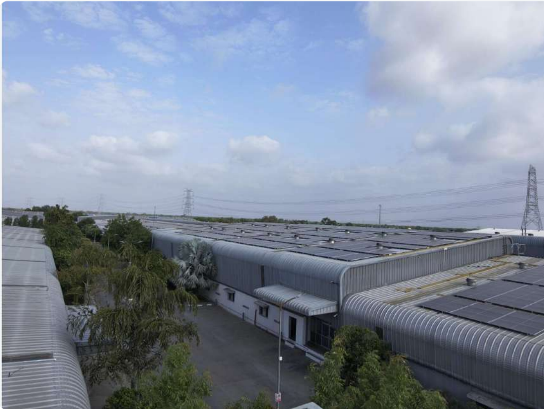
Texspin's clean-energy footprint — rooftop and ground-mounted solar integrated with the grid.
